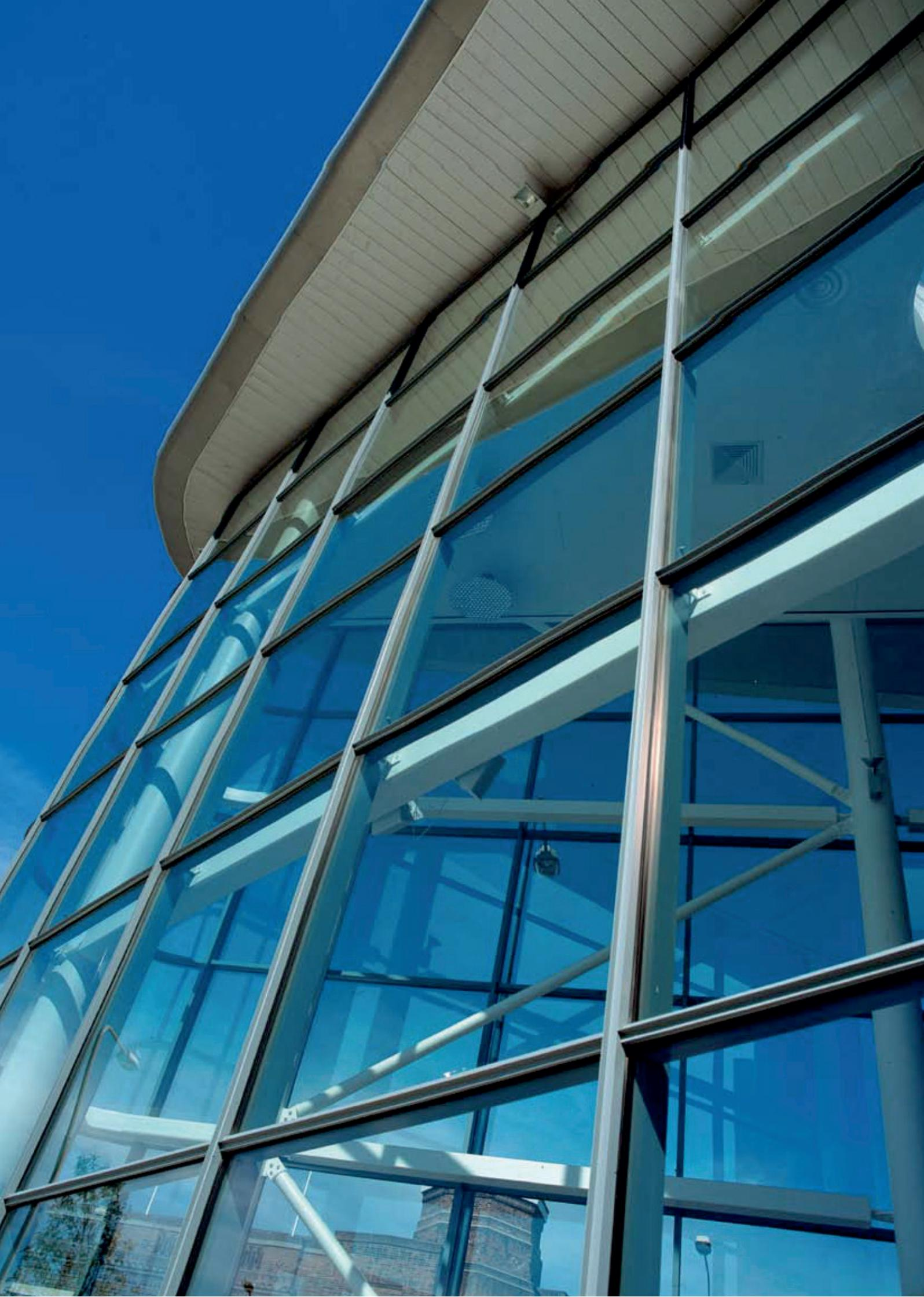
Elegance 52 is a comprehensive curtain wall system that combines technology and design with the demands of contemporary building design and construction. All Elegance 52 systems use a common substructure with a width of 52 mm, allowing a slim sightline, whilst maintaining the necessary strength and inertia requirements for most applications.
